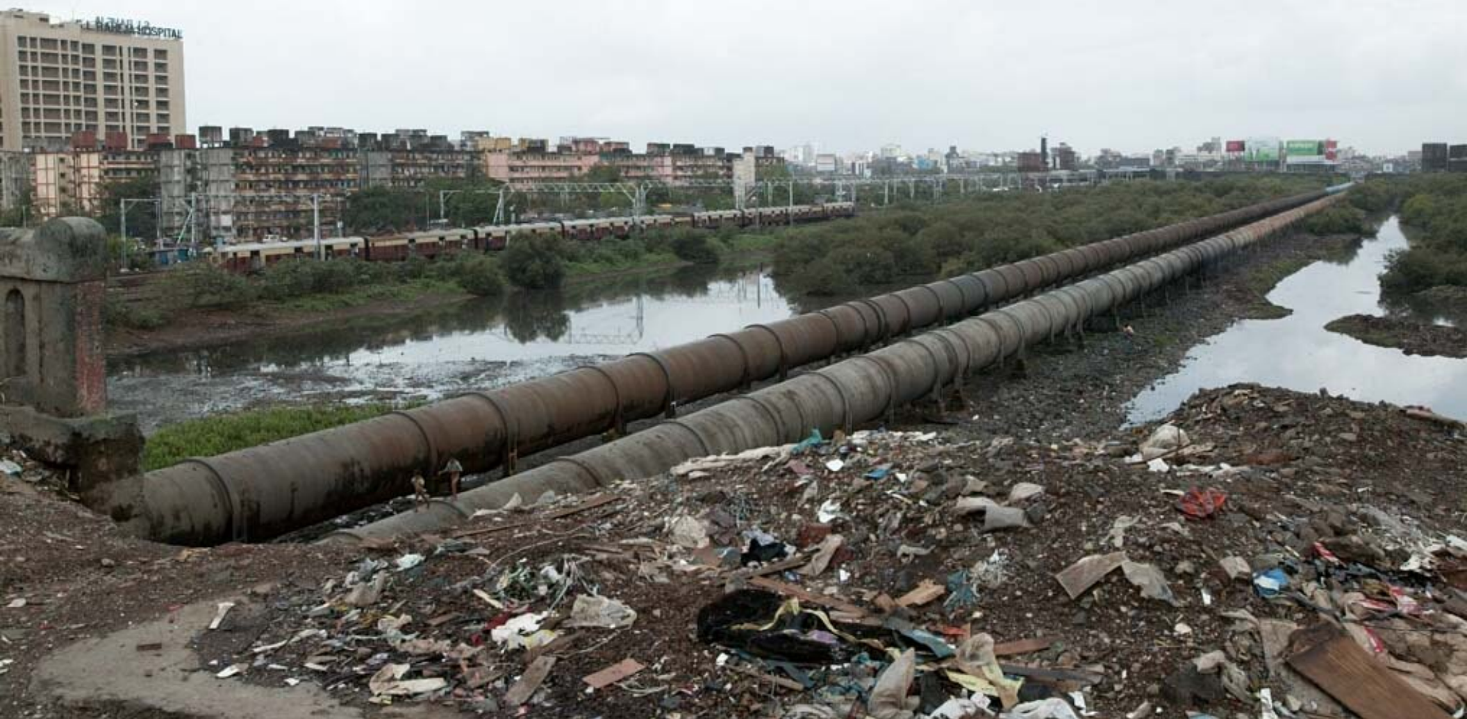
DESTRUCTION OF MANGROVES
